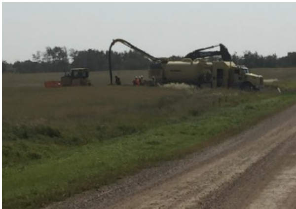
Hydro vac bore hole – km 14+100 – Aug 21, 2018
