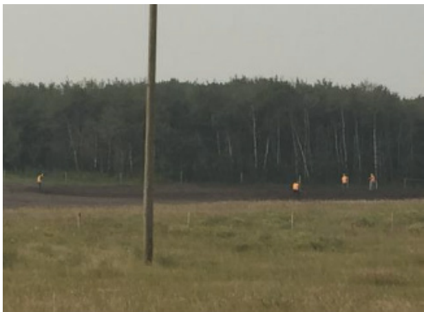
Utility crew picking rock and wood debros– km 17+500 – Aug 23, 2018
