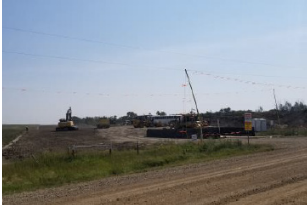
Dozer being cleaned – SF 18 – Aug 21, 2018
