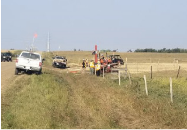
Crew building fence – SF 3 – Aug 25, 2018
