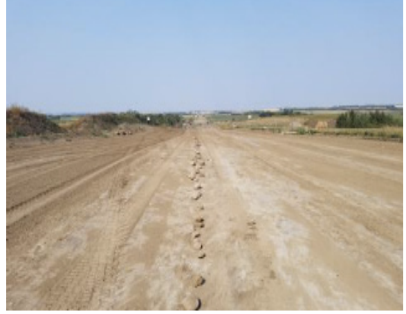
Crew rock picking – SF 21 - Aug 25, 2018
