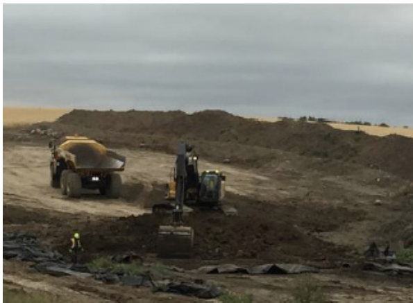
Excavator ramp removal – km 34+000 – Aug 24, 2018
