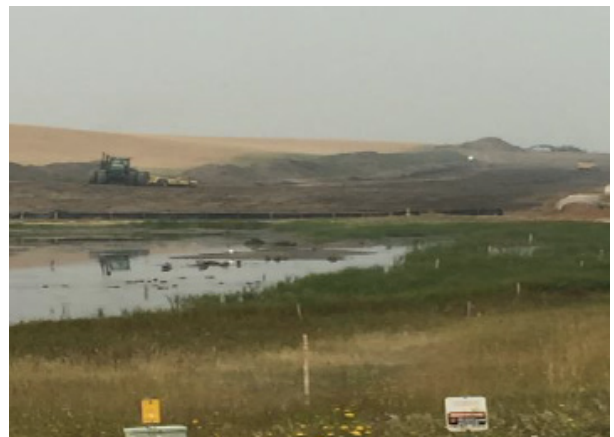
Discing and grading– km 108+650 - Aug 23, 2018
