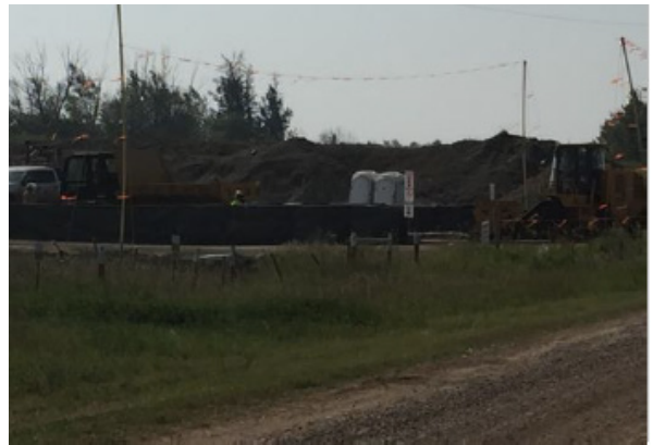
Silt fencing, Ribstone Creek– km 37+750 – Aug 21, 2018
