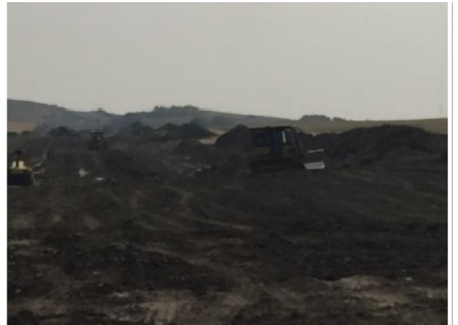
Grader and dozer – SF 21– Aug 25, 2018
