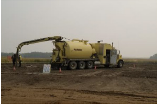
Hydrovac daylighting pipe – SF 10 – Aug 23, 2018
